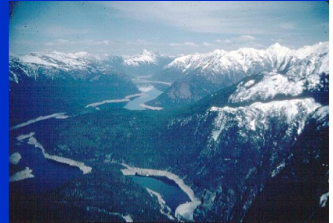
Skagit River Hydroelectric Project - Ross Reservoir
